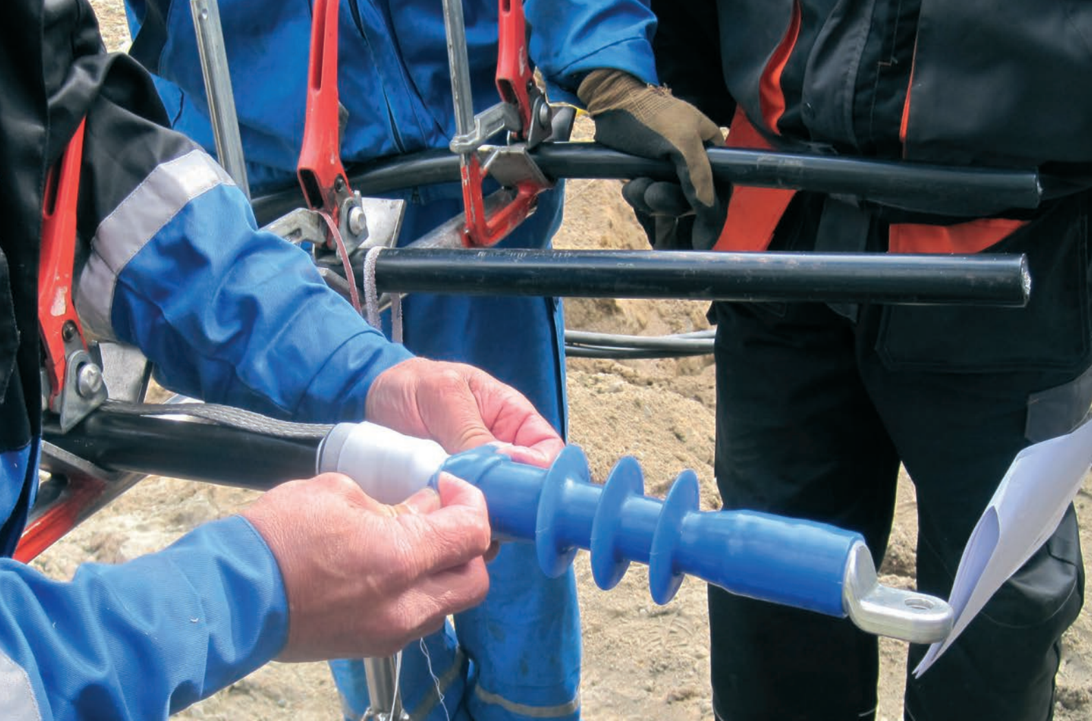
Cold shrink joints dramatically reduce failure rates.
